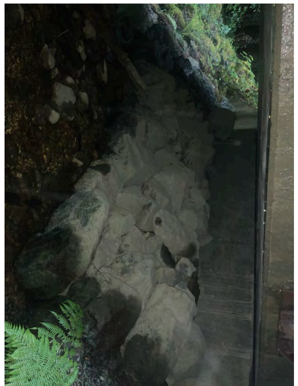
Right Bank Abutment when facing downstream
